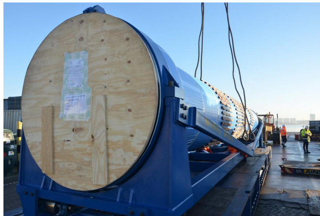
Autoclave: Arrival at Walton facility
