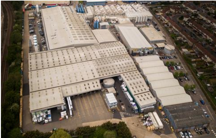
Croydon, UK: largest site, AZOTE and all HPP foams
